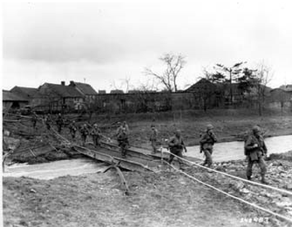
Figure 65 Treadway bridge over the Erft at Bliesheim
