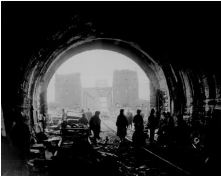
Figure 72 Remagen view from the tunnel
