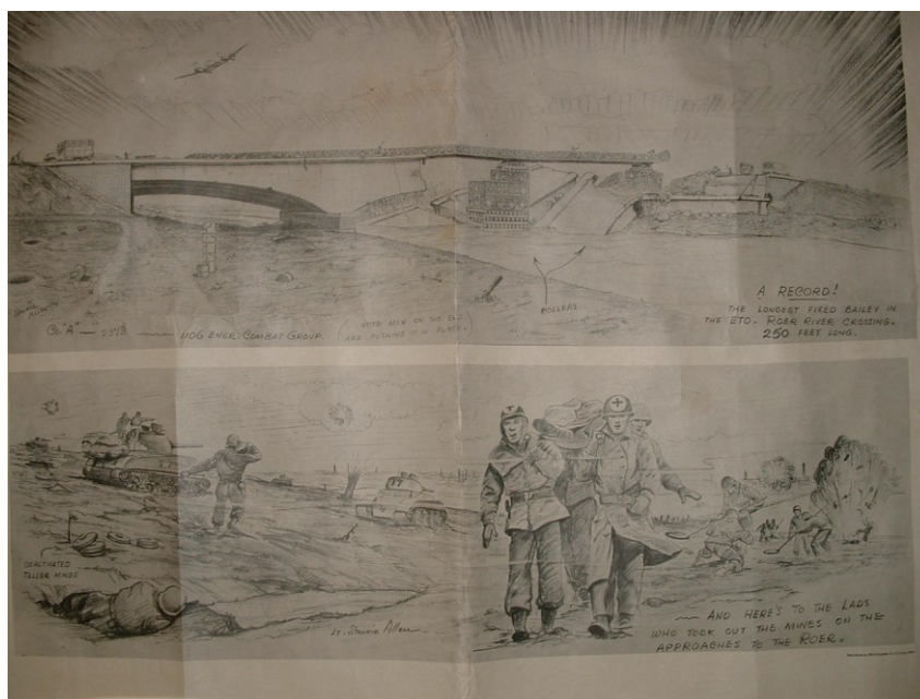
Figure 52 Crossing the Roer
